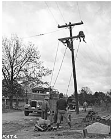
REA Photograph: “Stringing Rural TVA Transmission Line”
