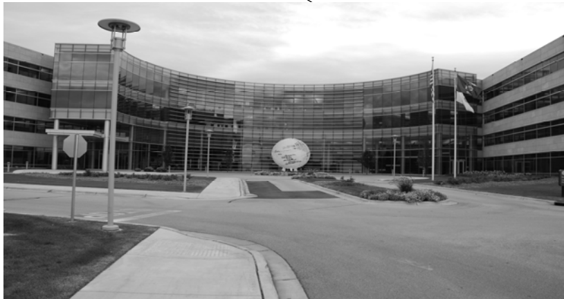
Lemberg Electric Company, Inc. GE Research Park - Milwaukee, Wisconsin
